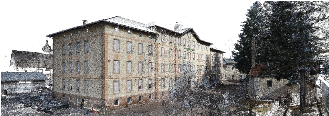
Figure 2: View of the point clouds from the survey of Macchi barracks
