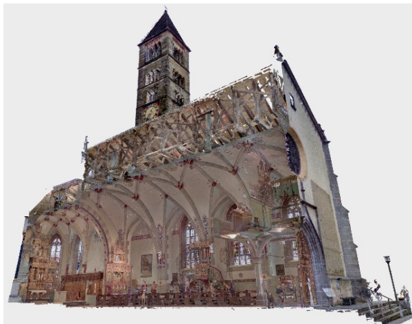
Figure 3. San Vittore Mauro Church at Poschiavo: view achieved by laser-scanner points cloud
