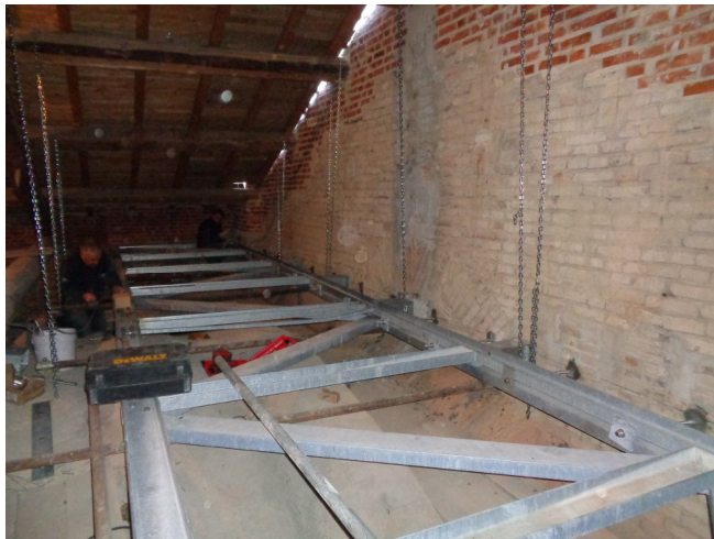
Figure 8: horizontal metal truss of the front façade Figure 9: Pull-out test on the connectors with the façade
