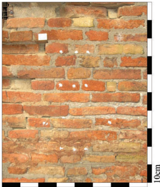
Figure 1. Texture of traditional brick masonry of Emilia region.
