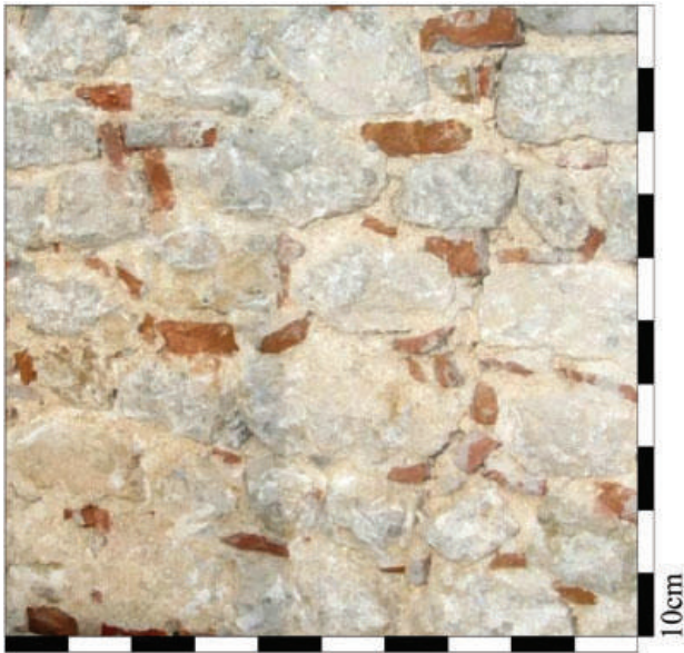
Figure 8. Texture of traditional brick masonry of L'Aquila historical centre.
